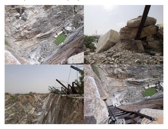
Prima facie cause of the accident : The accident was occurred due to fall of side (common boundary between QL No. 167 and 168) having height of about 10-15 m. the side consisted of fractured/jointed rock.
